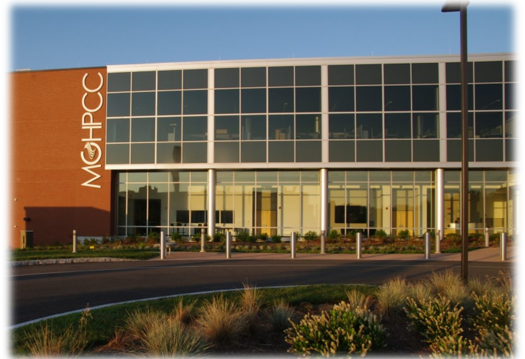
MGHPCC: Massachusetts Green High Performance Computing Center
